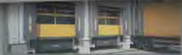
Refrigerated distribution centres
