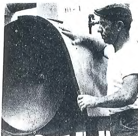
Armaflex II Sheet is always applied with the smooth side out. It is easy to cut to fit around piping or projections.
